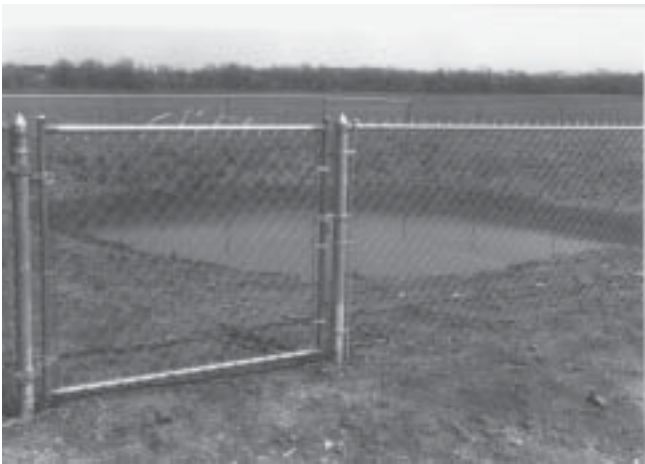
Figure 3. A fine new wastewater pond. This chainlink fence will have a long life and requires little maintenance.
